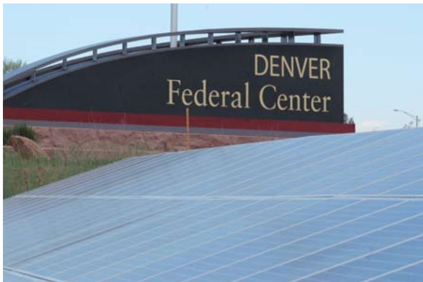
The Denver Federal Center will install roof-mounted solar panels that will save over $300,000 in electricity per year.
